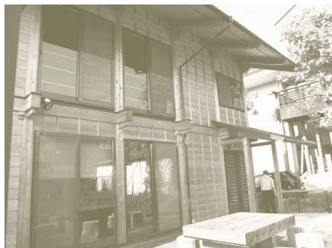
Experimental timber house in Kyoto University
