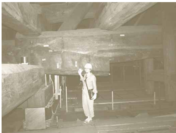
Roof timbers in Kyoto temple
