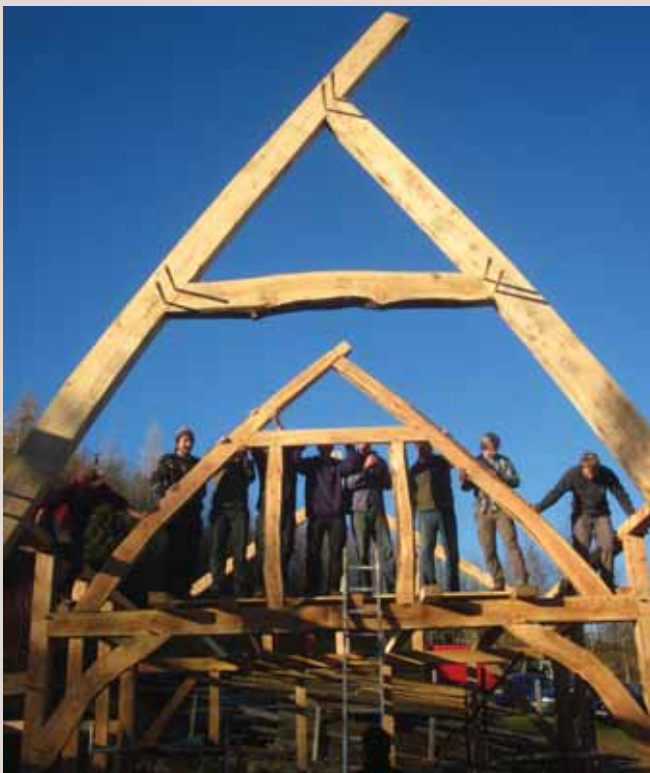
Erecting the workshop frame
