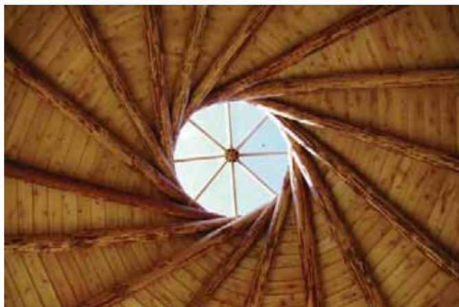
The reciprocal roof of the Roundhouse at South Harting School.
