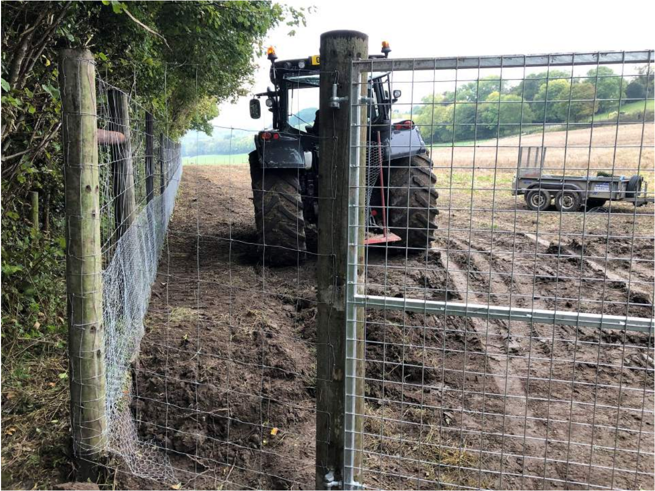
Figure 11 Fence erected at Fontmell.
