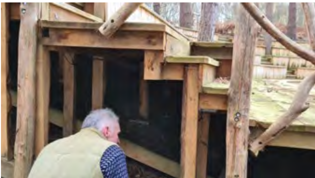
Mark inspects the Chestnut stakes supporting the seating
