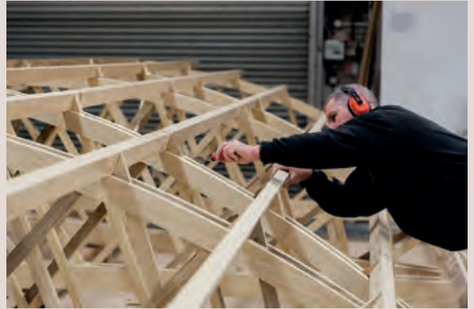
Built: East Pavilion by OGU Architects + Donald McCrory Architects
