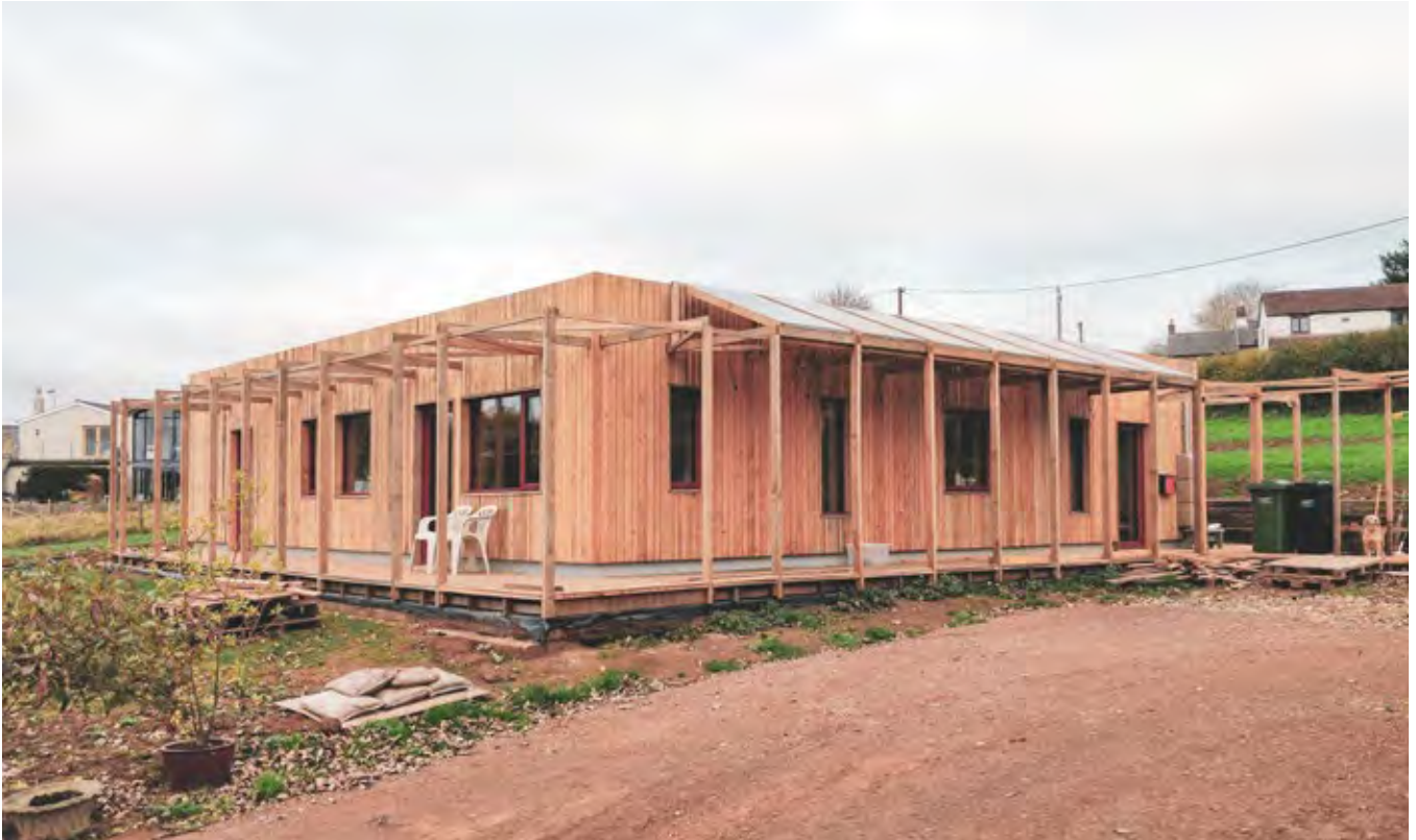
Nest House nearing completion
