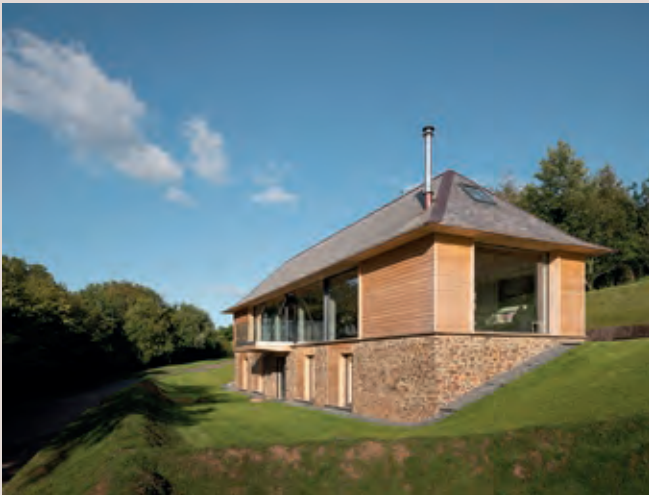
The Boathouse by Adams Collingwood Architects
