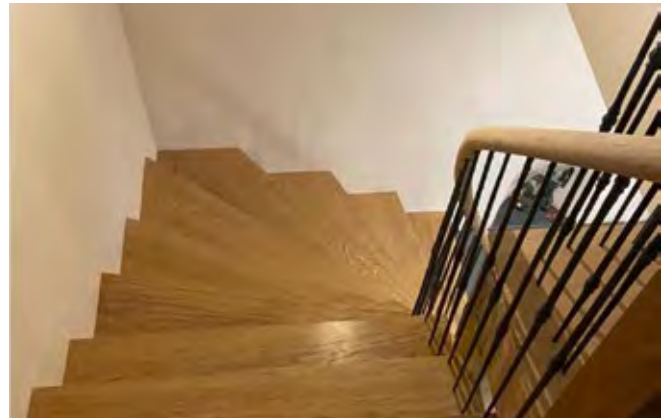
Oak curved kite staircase by Woodfellows Joinery
