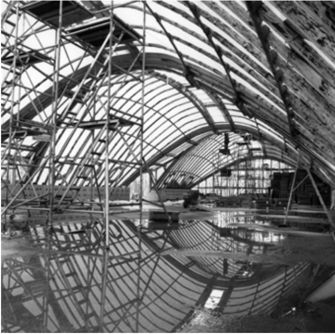
Designed by Richard Burton of ABK and Frei Otto, with the engineers Buro Happold, Hooke Park's main workshop is an impressive long-span enclosure built using low-value material from the surrounding forest. Completed in 1989
