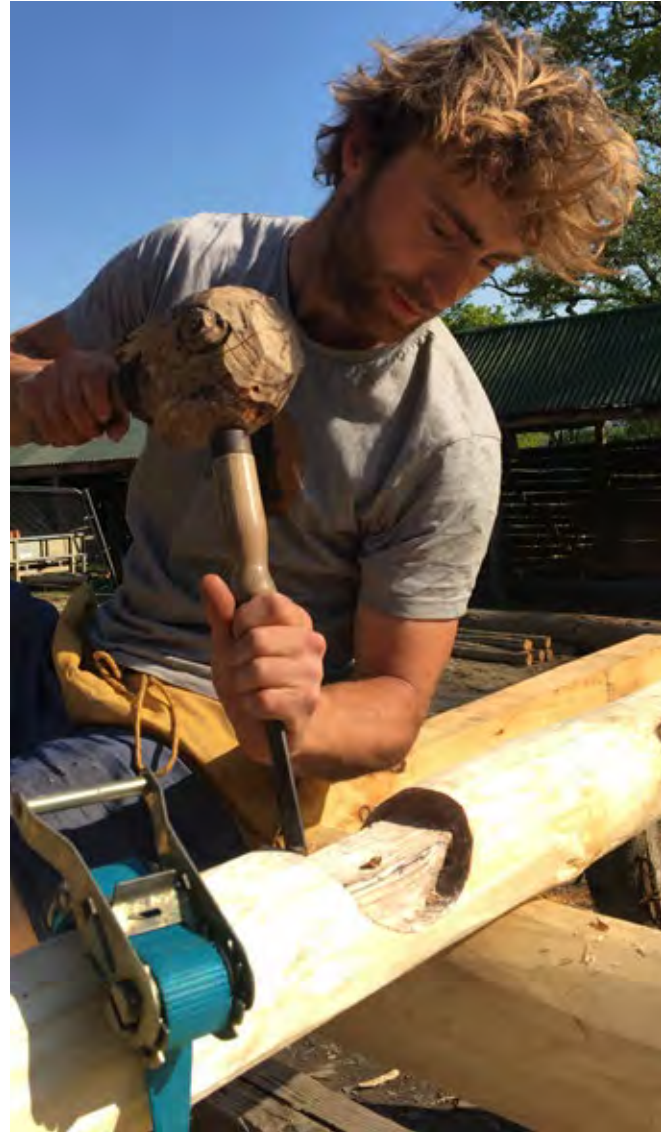
Making a butter pat joint
