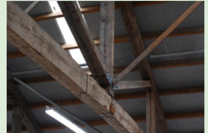
Corsican Pine roof beams
