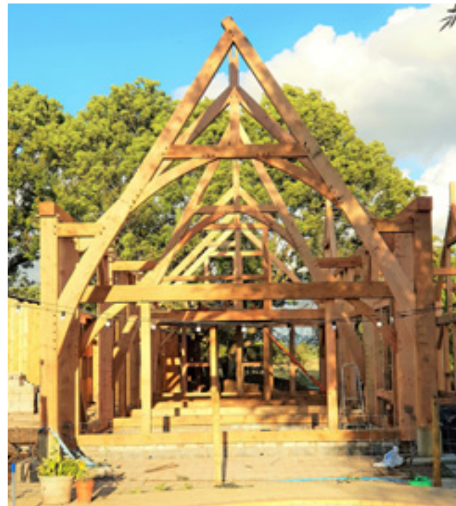
Timber frame for a four-bed, two-storey house in Preston
