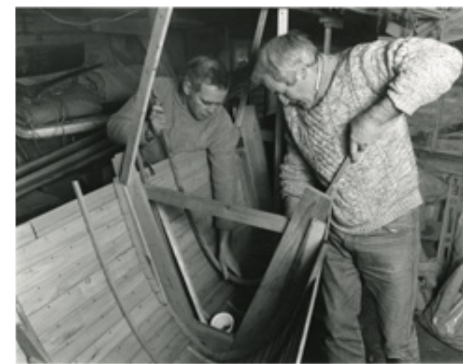
Construction of William Peters - fitting a steamed rib
