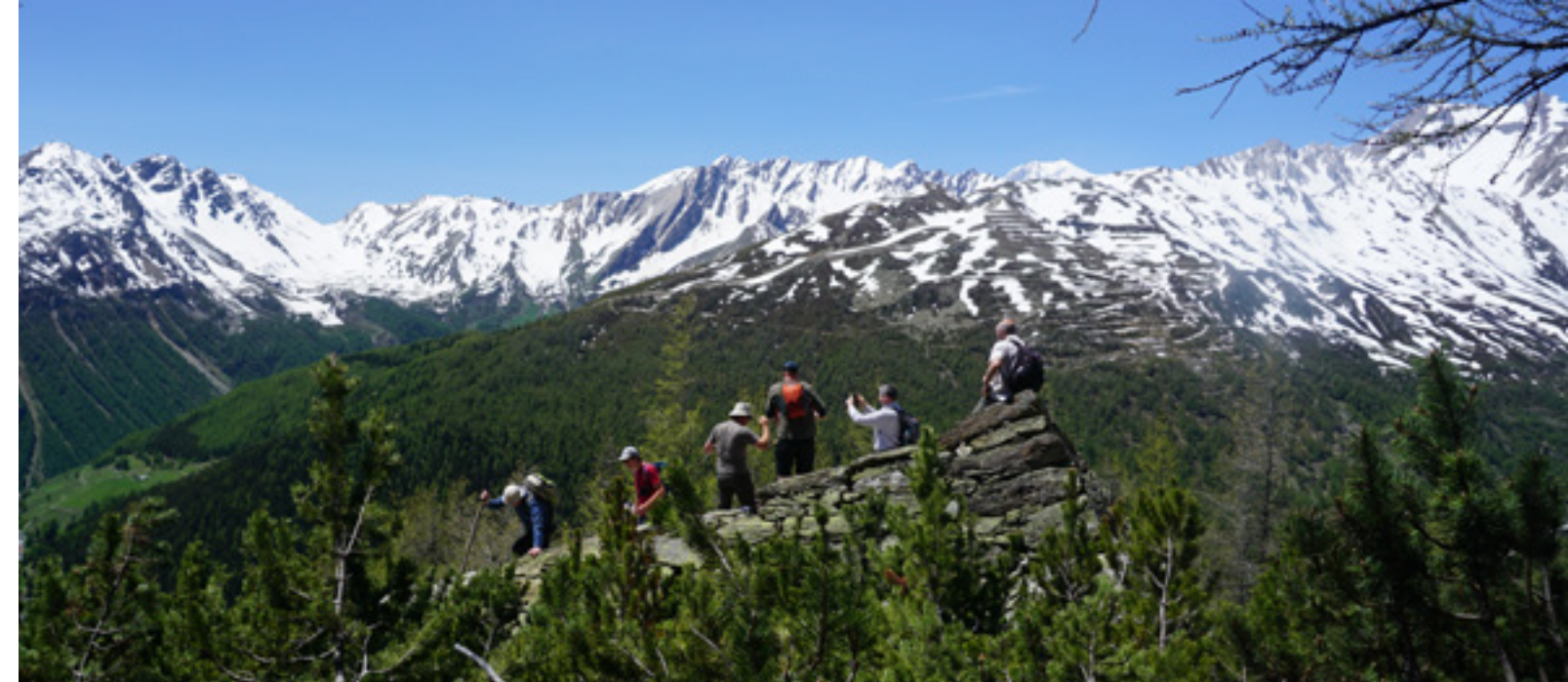
The group viewing the local landscape of high alpine peaks, forested lower slopes and valley bottoms laced with roads, railway lines and villages from a stone avalanche defence built in 1841. Forests provide a key protective function, slowing and catching avalanches and rock falls
