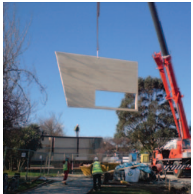
Falmouth School – Speedy assembly of the pre-cut cross laminated timber panels
