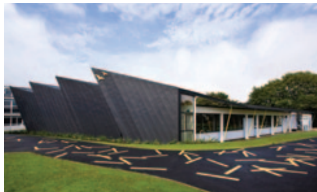
Falmouth School – Speedy assembly of the precut cross laminated timber panels
