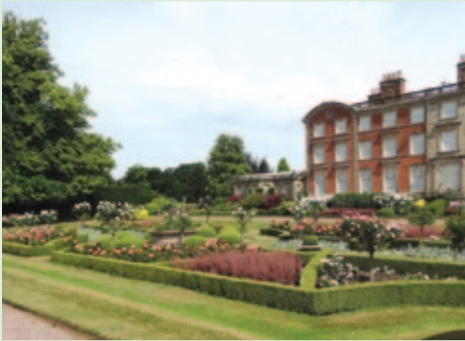
The south facade of Weston Park
