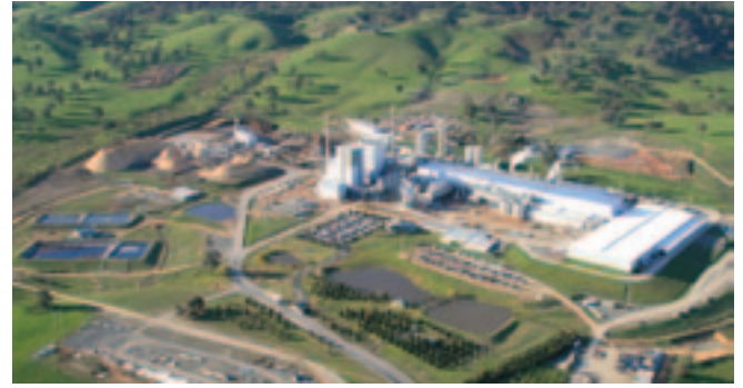
Australian plantations now supply fibre for world-class pulp and paper investments such as Visy's $1.1 billion plantation-based Kraft pulp and paper mill at Tumut, New South Wales
